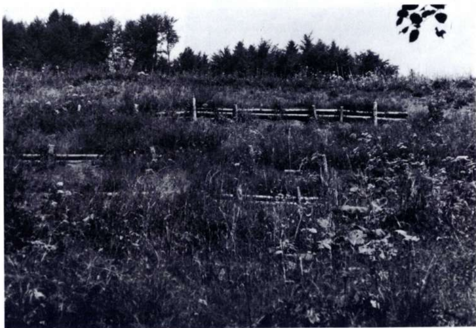
Fig. 2 - Dissesto quasi completamente bonificato tramite fascinate. - Landslide almost entirely reclaimed with fascines.
